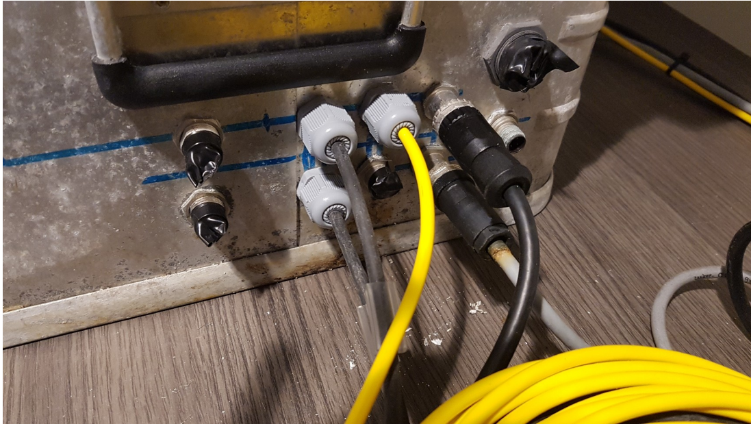
Figure 7 – The new cabling – external connectors (April 2023)
